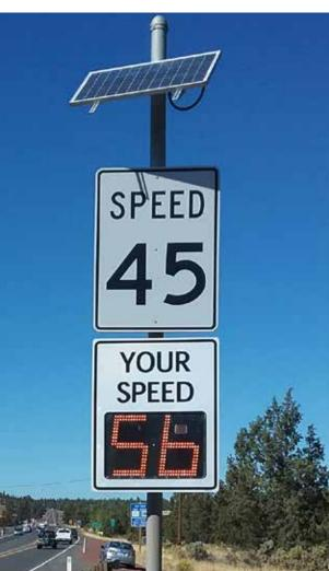
5 Solar-Powered Speed Radar
